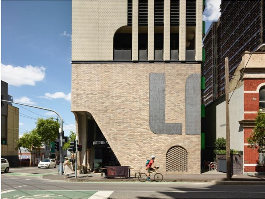
Within the podium, deep concrete lintels accent the brick and provide another nod to the concrete and bluestone lintels of times gone by. Immediately above the podium, tessellated precast concrete panels reference the textile and boot maker industries with their woven, textured appearance, adding an almost fabric feel to the building's skin, while their complex patterning delivers a
